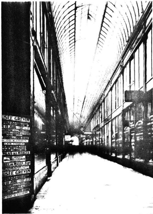
59. SKYLIGHT REINFORCING SPINE
