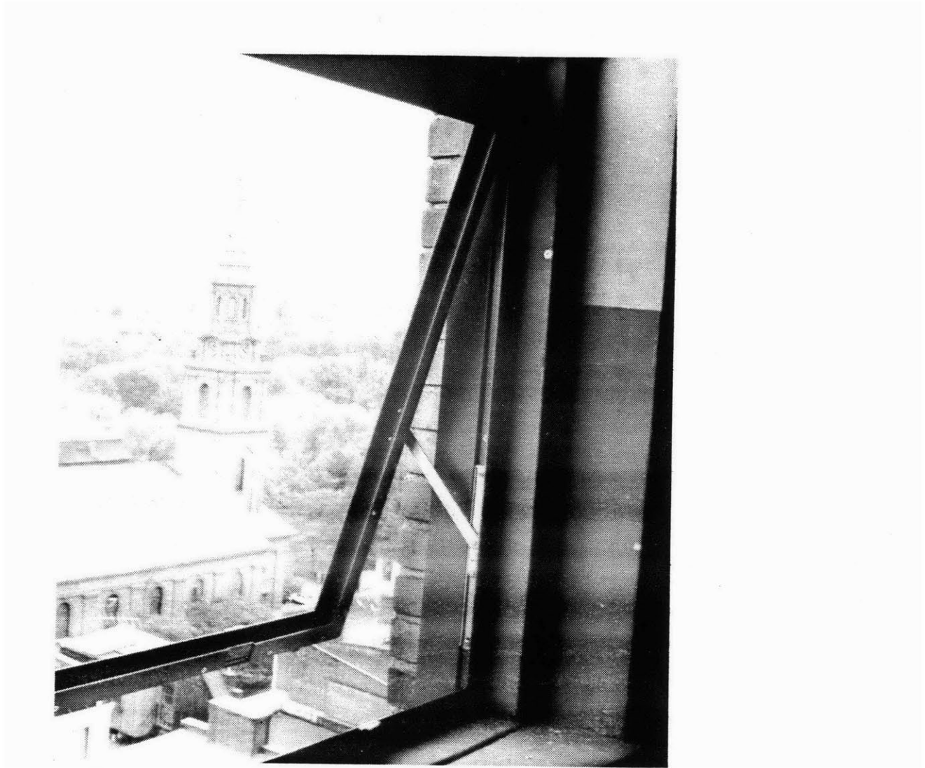
Awning Window, as installed
