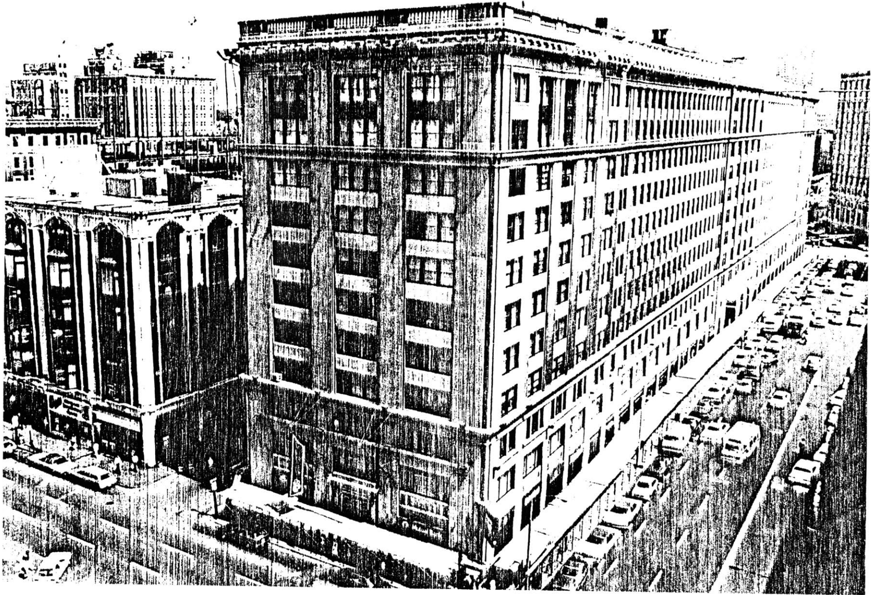
The Park Square Building before cornice removal.
