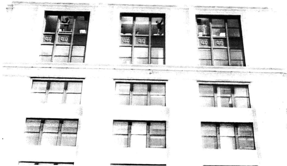
• Installation of the new window units on the 11th floor, Berkeley Street end, mid-November, 1984.
