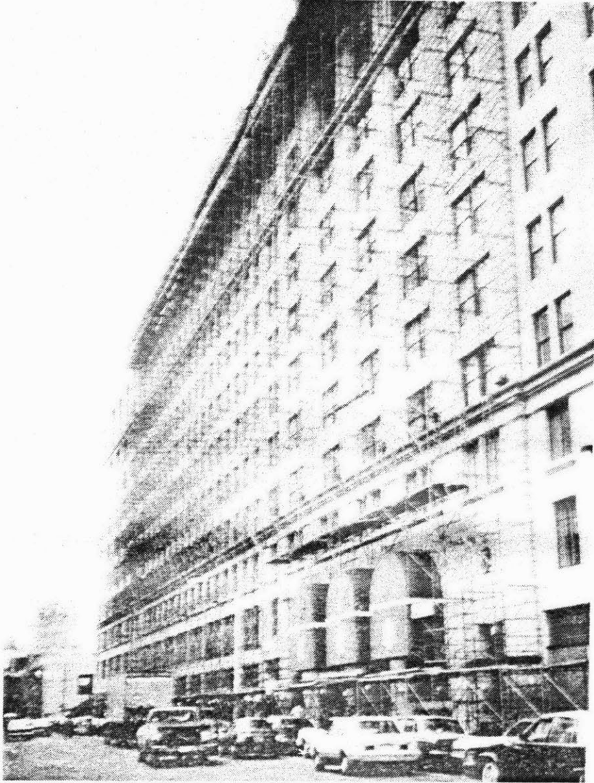
Scaffolding on the St. James Avenue Facade
