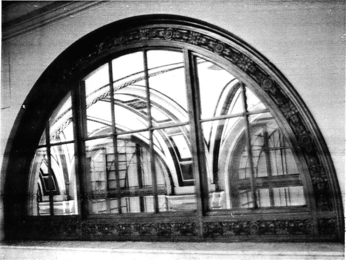
View from 2nd Floor Lobby into Main Entrance Vestibule
