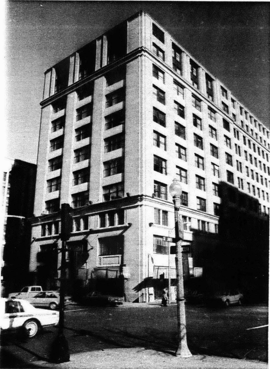
Park Square Building from the corner of St. James Avenue and Berkeley Street
