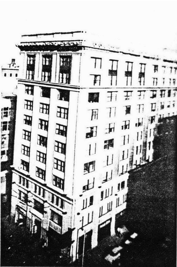
The Park Square Building with parapet
