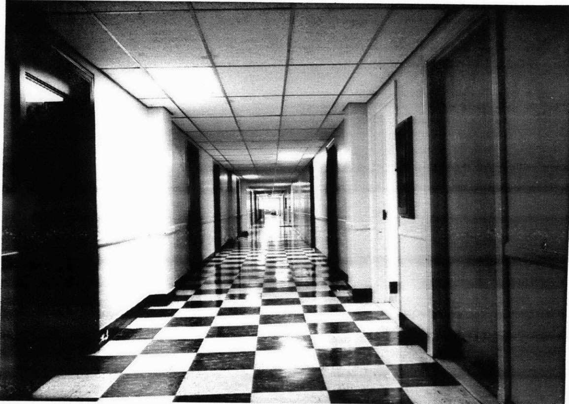
Typical tenant corridors prior to renovation
