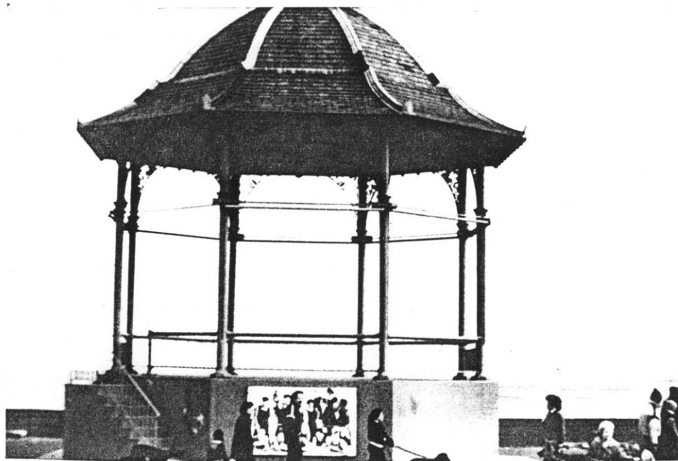
Closer view of bandstand built for Olmsted's turn-of-the-century beachfront promenade.
