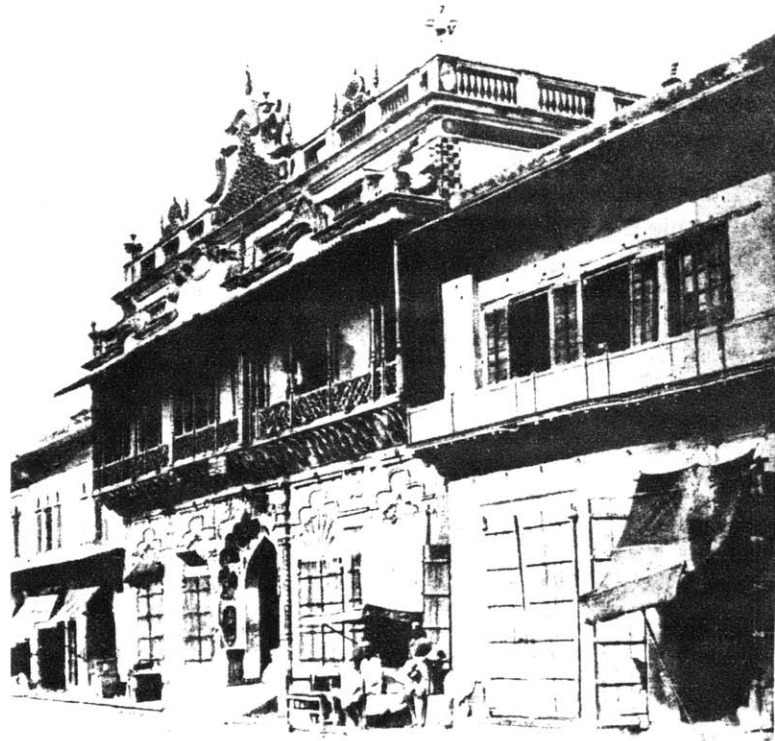
Fig.4.2.6 The articulation of facades on the main thoroughfare, Chandni Chowk. The ornate design, the awnings shading merchandise and people on the sidewalks, and the pavement life.
