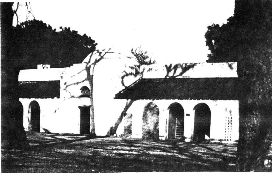
Fig.6.4.1 Govt. housing for clerks in New Delhi, designed by W.H. Nicholls in the immediate post-Lutyens era.
