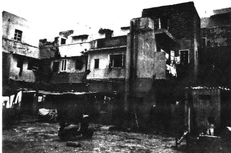
Fig.6.4.2 Refugee resettlement housing built in the forties and early fifties, showing the richness they have come to manifest as they age over time.
