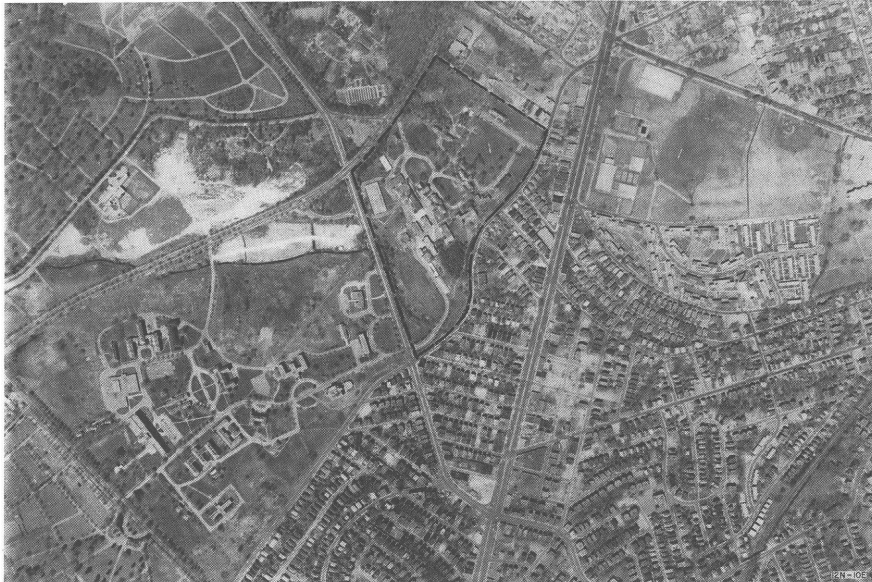
Aerial photograph of site
