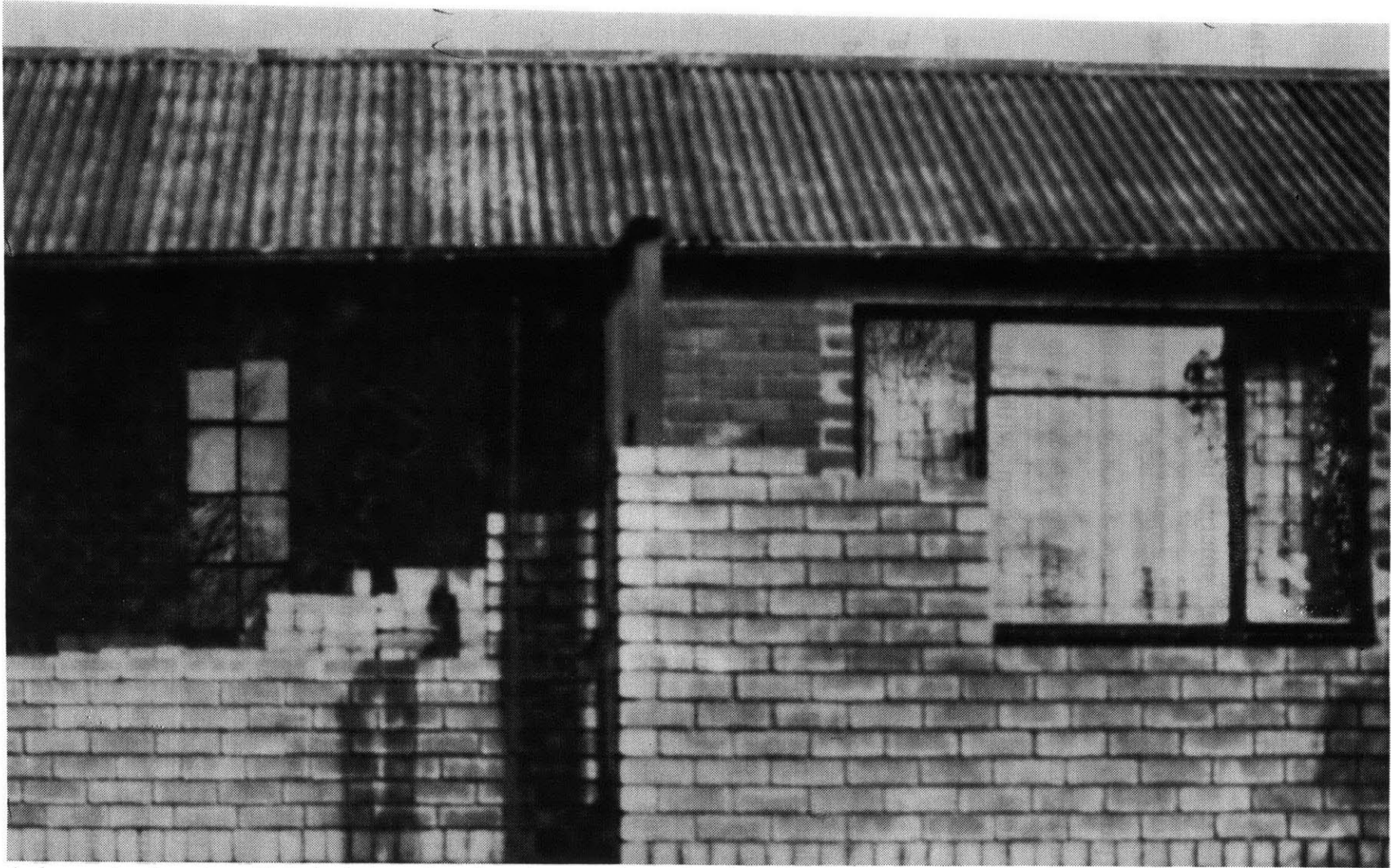
A house in Soweto which is being altered and a porch enclosed. The large window on the right also appears to be an addition.
