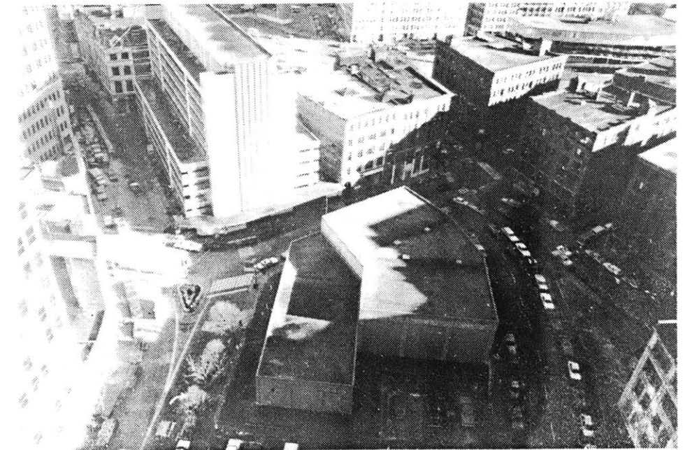
View of site from Lafayette Place.
