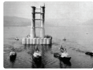
CONDEEP PLATFORM TEMPORARILY FLOATS BEFORE OIL RIG CONSTRUCTION
