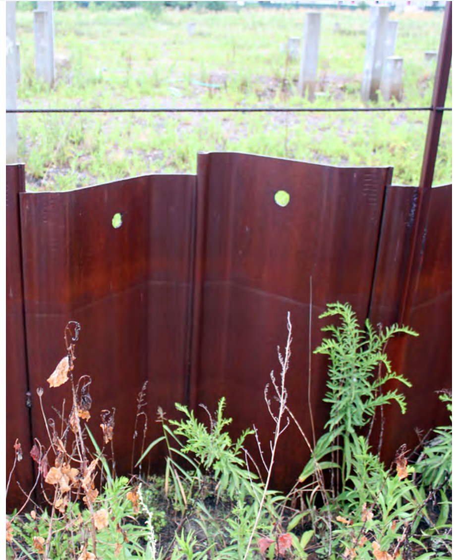
Figure 31. East Boston, Pier 01 Site, Steel Plating
