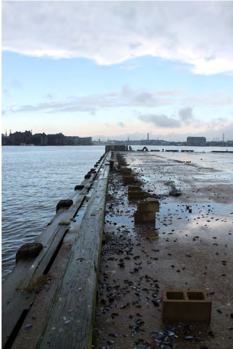
Figure 30. East Boston, Pier 01 Site, Hard Water's Edge
