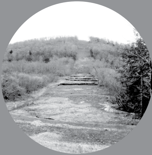
CLEAR CUTTING FOR PIPELINE
