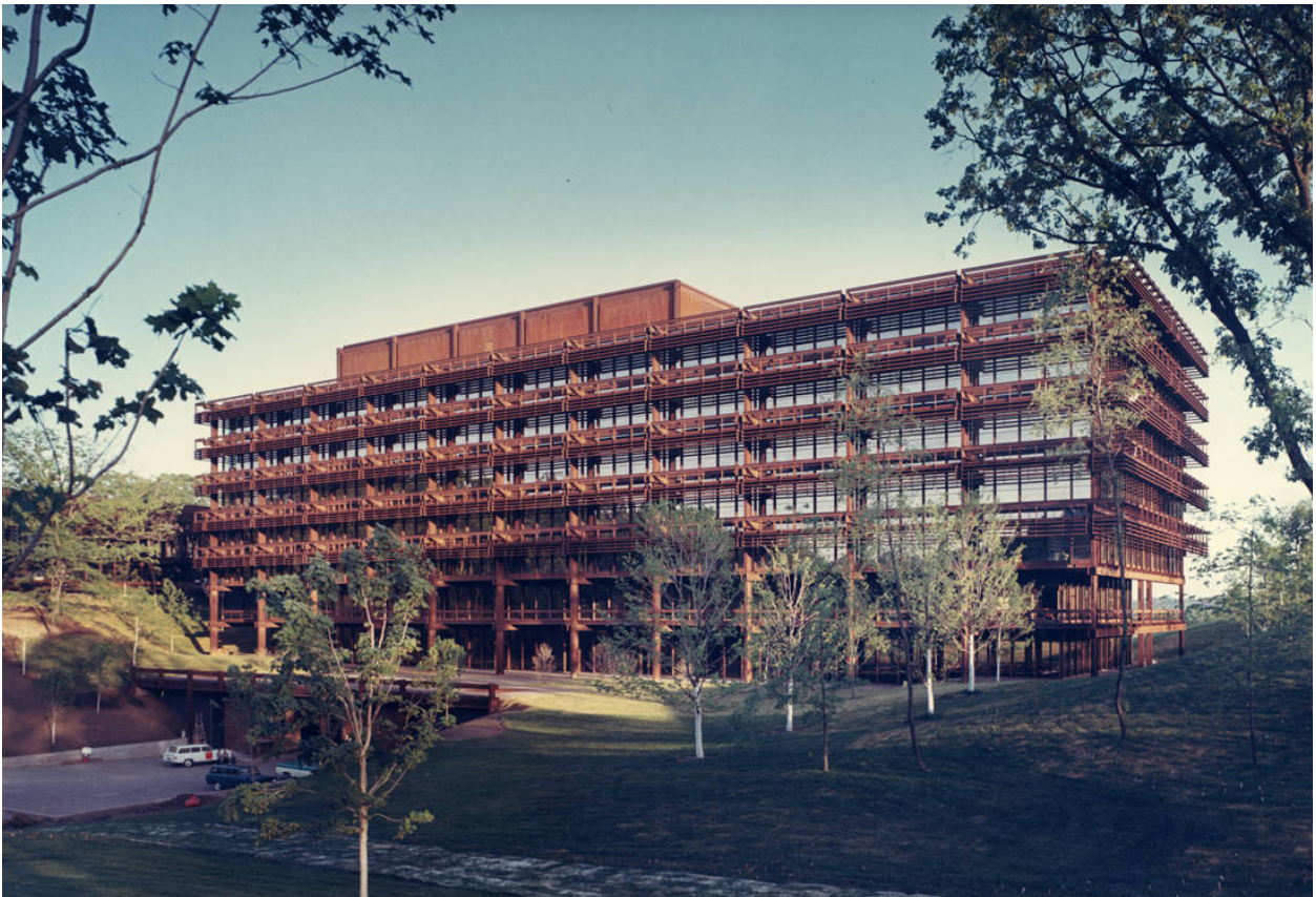
Figure 01: Deere & Company World Headquarters. Moline. IL. Source: http://architecture.about.com
