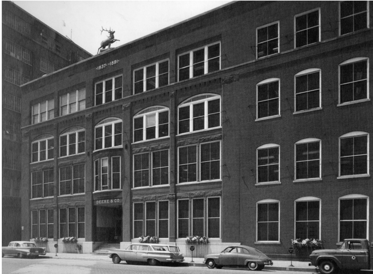
Figure 17: Historic Deere & Co Headquarters. Source: Mozingo 2011.
