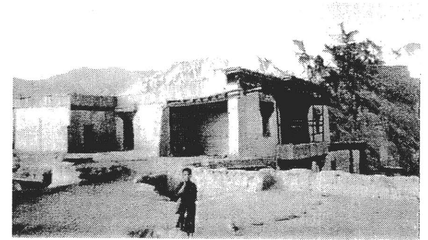
Fig. 28: The roof as an elevated plan
