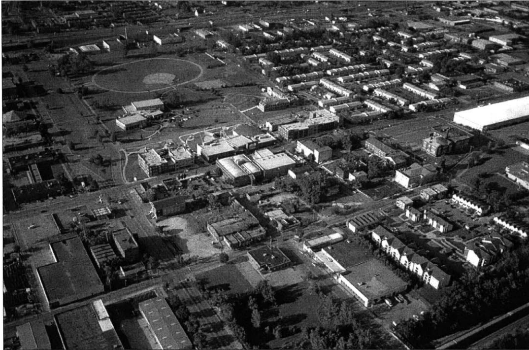
Figure 3.18. Aerial view, 18th and Vine Historic District (view northeast from Paseo Blvd. and Kansas City Terminal Railway). Interstate 70 runs east to west at the top of the photograph. The large development to the upper right is the former Attucks Housing Project. The grassy oval is the main ballfield in Parade Park. The Count Basie Court Apartments are visible in the lower right. Photograph by Alex S. MacLean, Copyright © 2002 Landslides Aerial Photography (used by permission).
