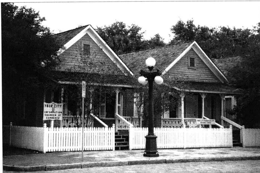
Figure 4.10. "Casitas" renovated by Tampa Preservation Inc., 1998. (Photograph by author.)
