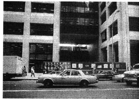
Regularly undergoing repair at 55 water street. Source: Kayden, p. 56.
