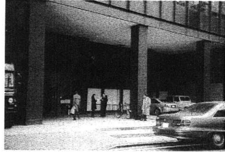
Cars parked in arcade at 160 Water Street. Source: Kayden, p. 57.
