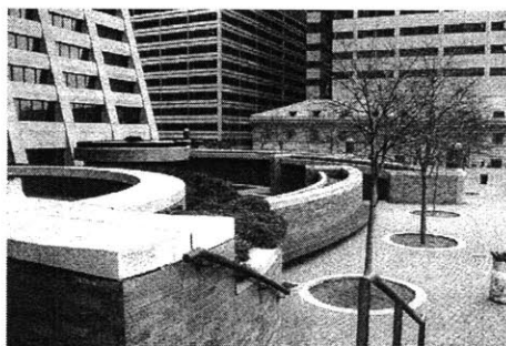
Elevated plaza at 55 Water Street. Source: Kayden, p. 36.
