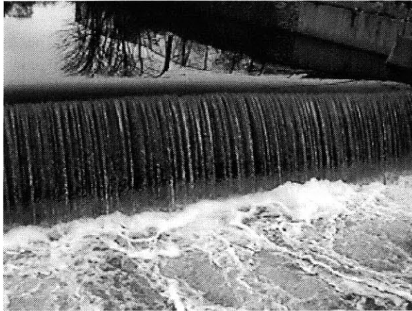
Figure 4-10. Route 85 Dam in Hudson
