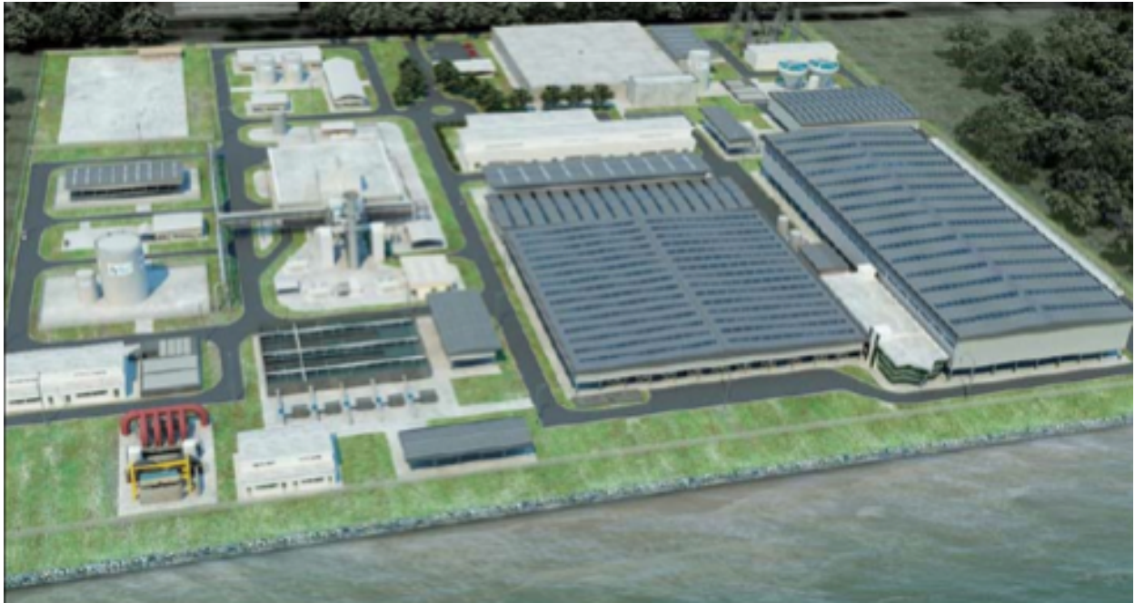
Figure 8: Aerial view of Hyflux's Tuaspring Desalination Plant (Hurn & Hagedorn, 2012)
