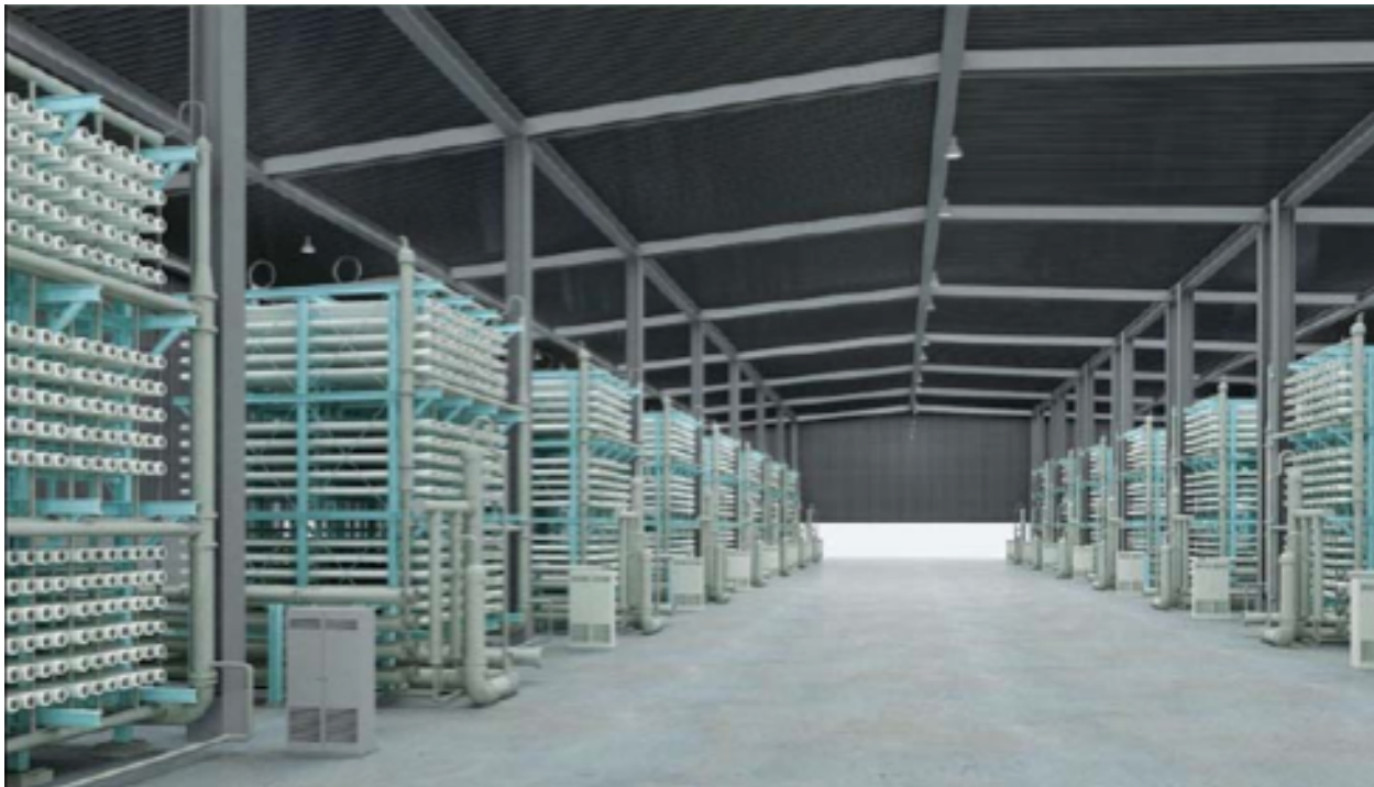
Figure 9: Interior view of Hyflux's Tuaspring Desalination Plant (Hurn & Hagedorn, 2012)
