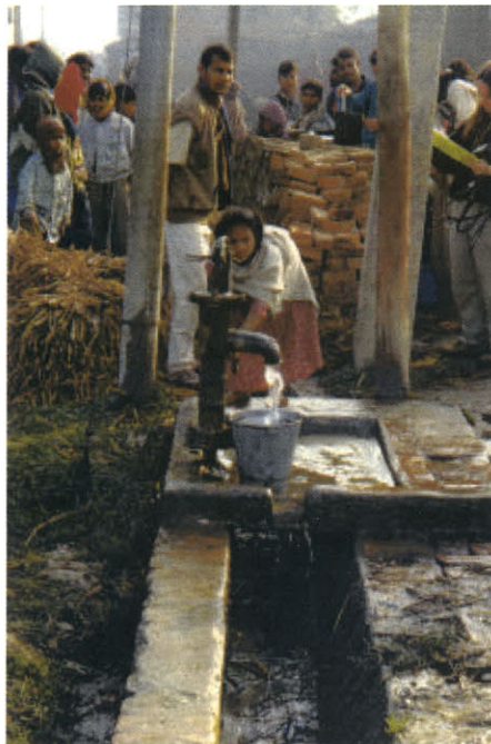
Figure 2.4: Sewer flowing adjacent to tube well in Birganj, Nepal
