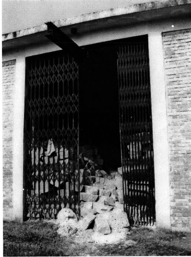
FIGURE 4-5: BULK ALUM STORAGE AT MAHANKAL WATER TREATMENT PLANT.
