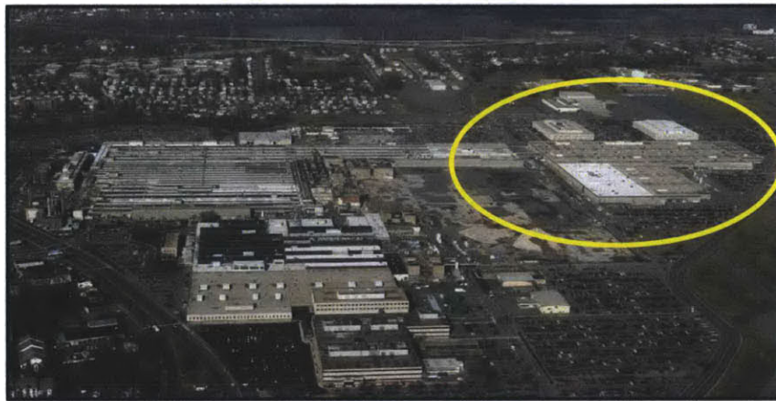
Figure 7: Overhead picture of the Pratt & Whitney facility in East Hartford, Connecticut. The circled building contains the Global Service Partners (aftermarket) division, including the Connecticut Stators and Components business unit and the Small Components Cell.
