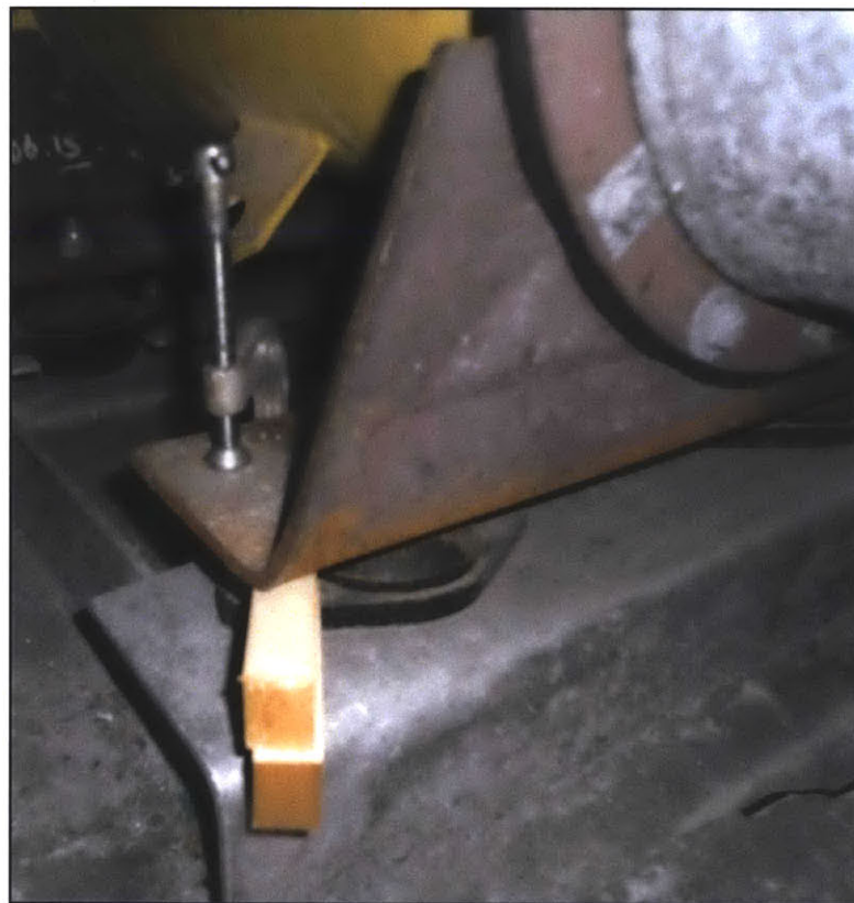
Figure 72: Clamped Mounts on SENECA Fans with C-Clamps and Wooden Blocks.
