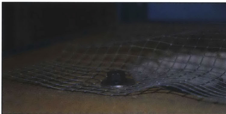
Figure 25: Tightened Mount on USCG Ventilation Fan [18].
