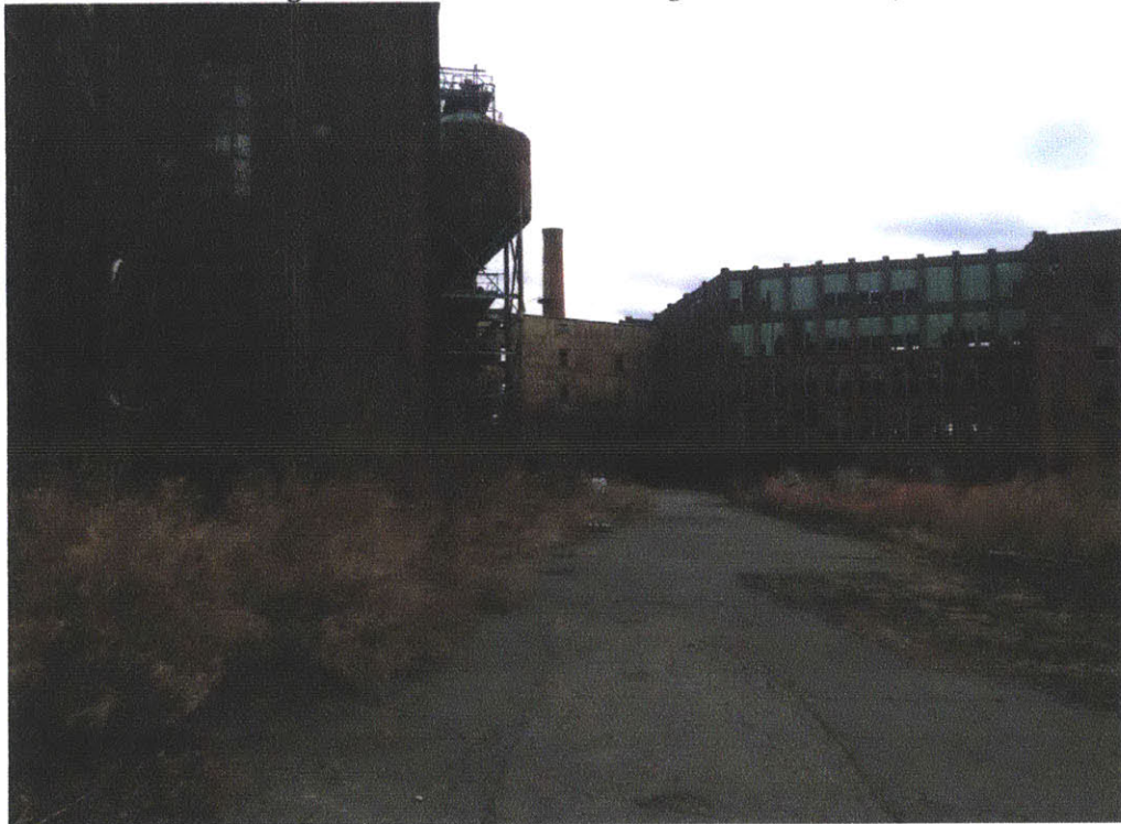
Image 2: Abandoned Buildings at the Uniroyal Site
