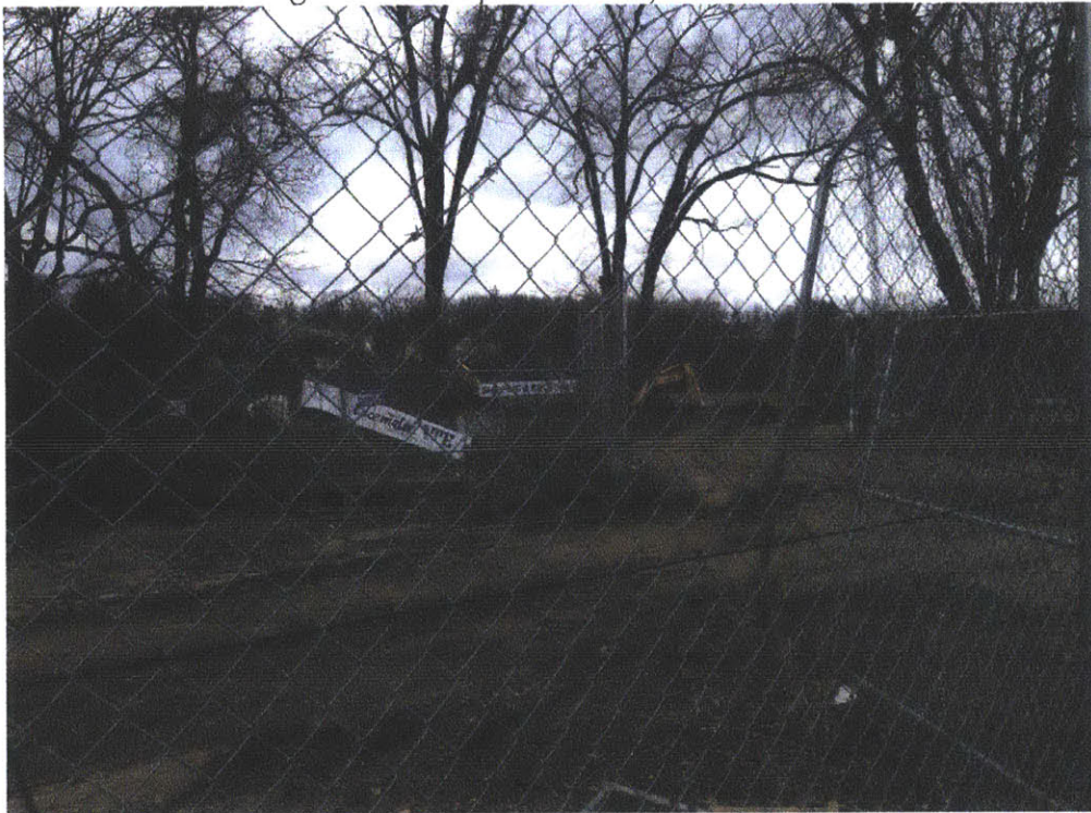
Image 1: Cleanup Underway at the Facemate Site
