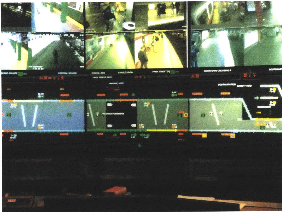
Figure 7: Real-time display of ATO information for the Red Line. The two parallel lines represent the tracks, and a red section indicates that a train is currently on that section of track.
