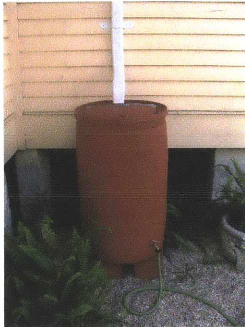
4.6 Typical Rainbarrel with Downspout and Spigot. Source: author
