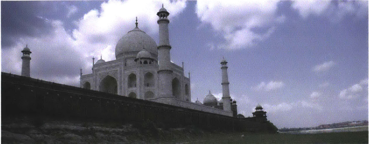
Figure 31 : Oblique View along Yamuna River
