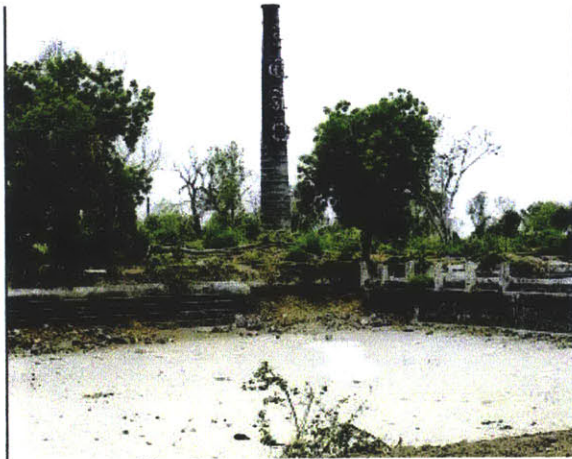
Figure 188 : The Calico Chimney
