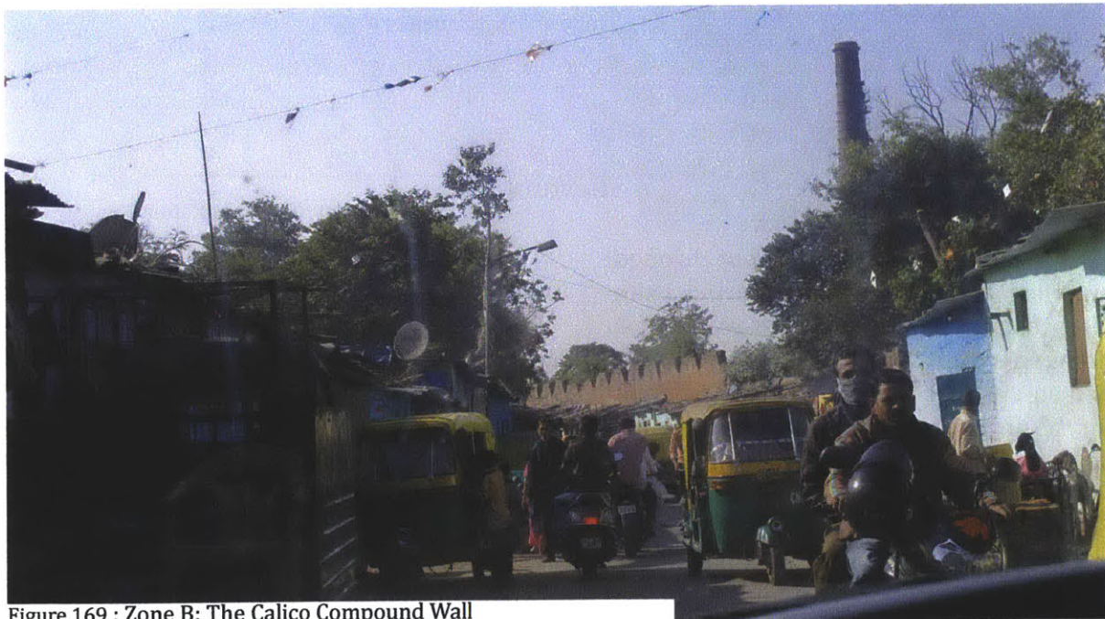
Figure 169 : Zone B: The Calico Compound Wall
