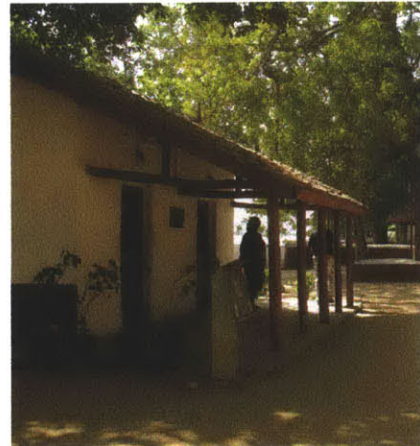
Figure 91 Simplicity in architecture Author . Site Visit January 2013.
