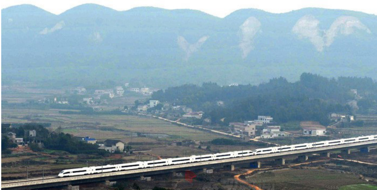
Fig 88. High speed rail crossing through the site - 2012
