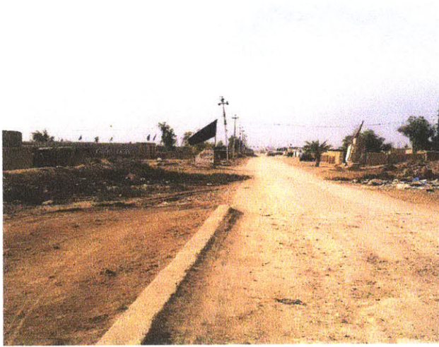
COMPACTED GRAVEL ON ROADS
