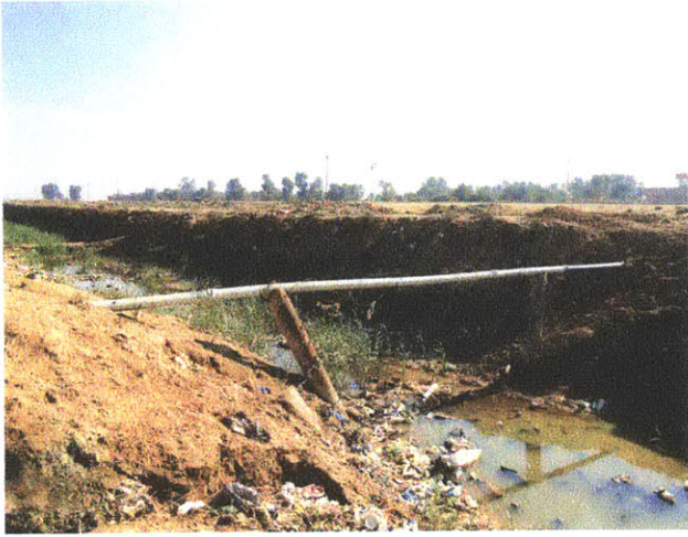
IRRIGATION CANAL ALONG SITE WITH STAGNANT WATER
