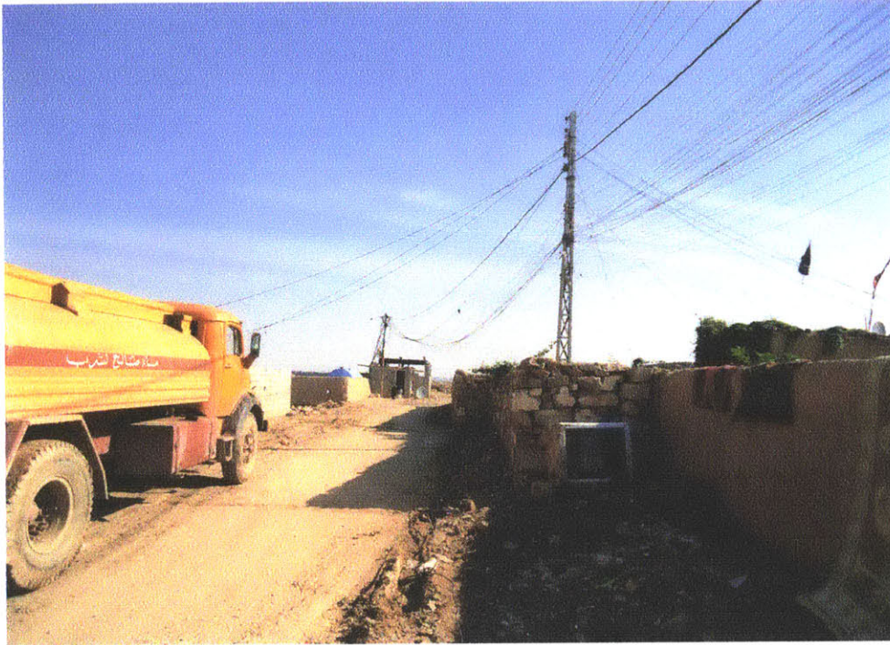
IMPROVED WATER SERVICES, ELECTRICITY, AND CONSTRUCTION
