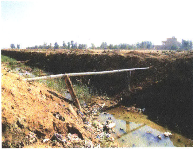
SALVAGED EXISTING WATER INFRASTRUCTURE
