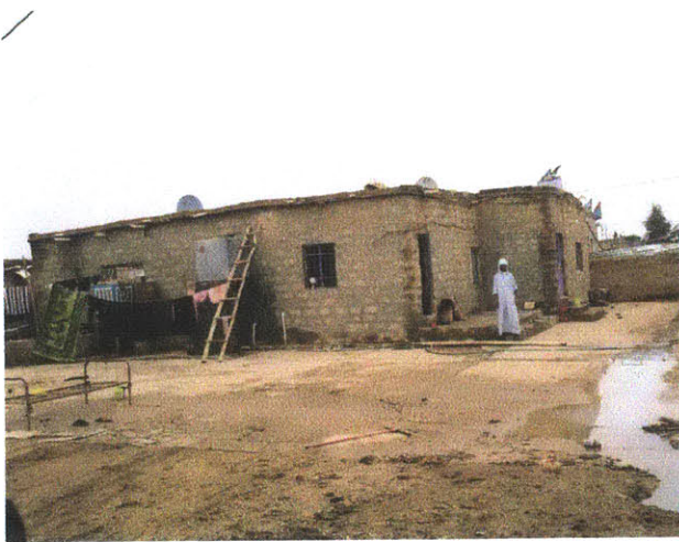
PERSONAL DRAINAGE CANAL
