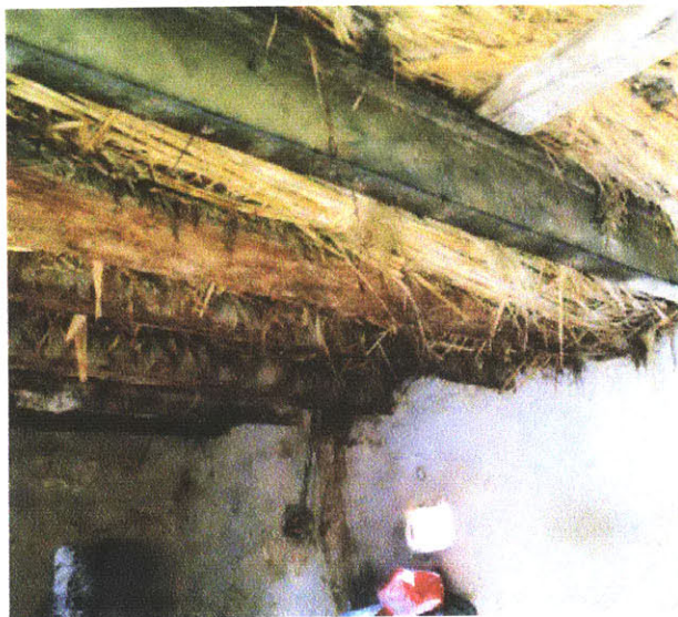
TYPICAL ROOF INTERIOR
