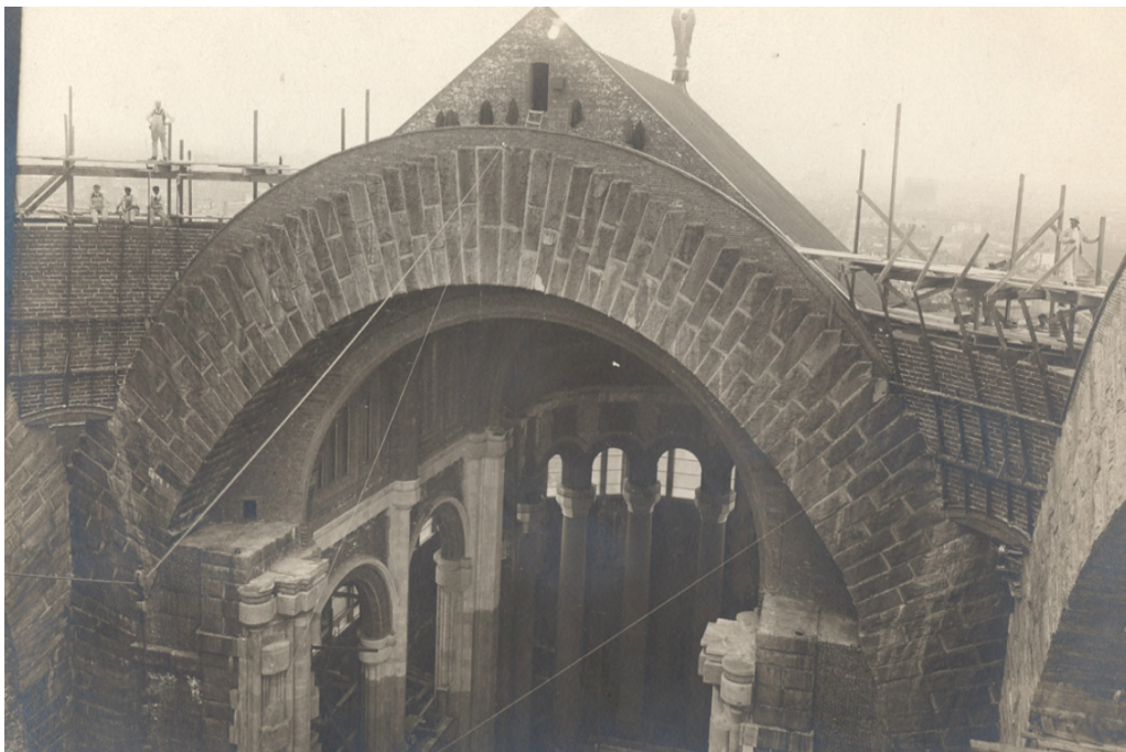
Figure 4.20: One of the supporting arches during construction [3]
