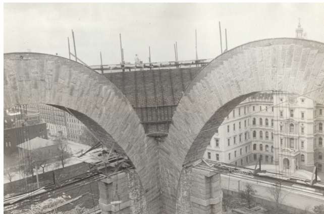
Figure 1.5: Pendentives of the dome under construction [3]
