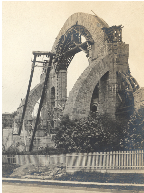
Figure 1.2: Construction of one of the great arches and its corresponding piers [3]
