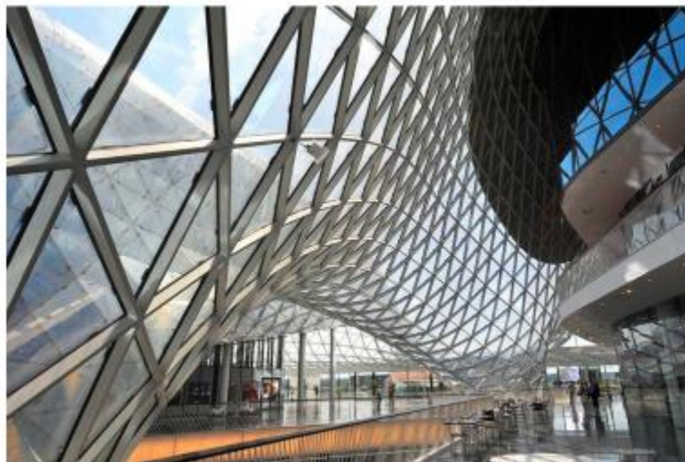
Figure 11: MyZeil Column-Free Interior
