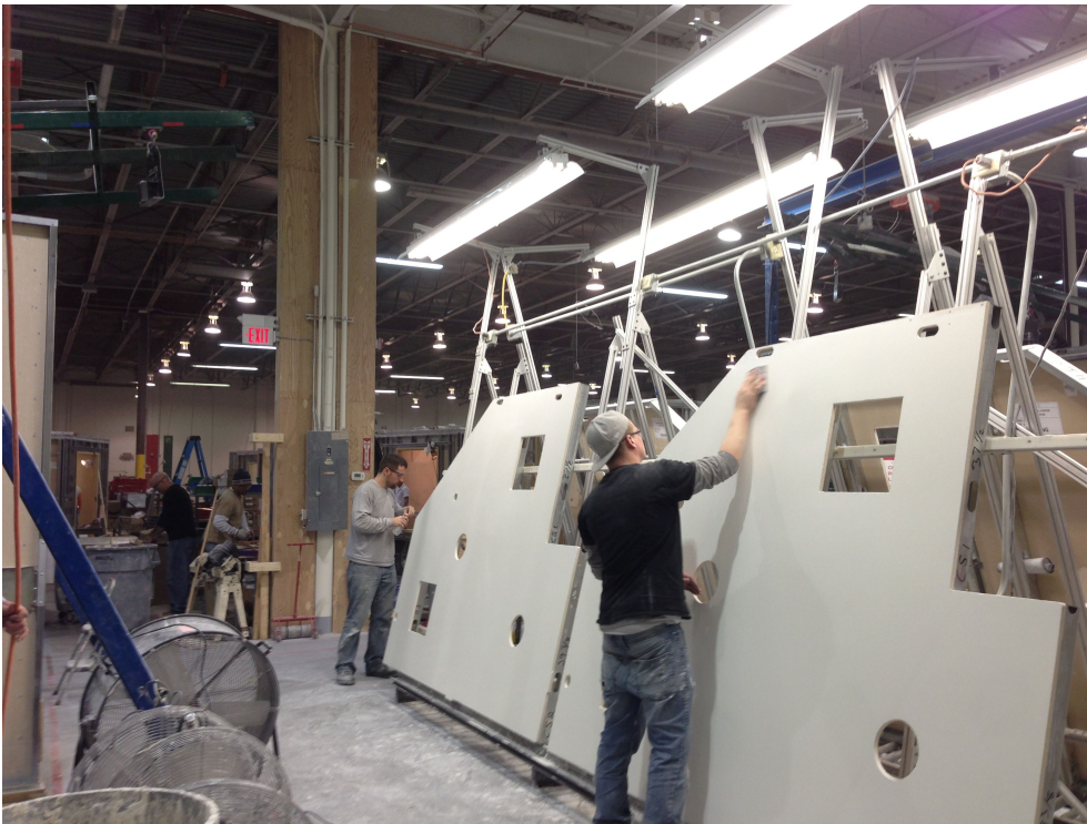
Figure 3.3-3: Workers perform tasks in a perfectly lit space (Eggrock Modular Solutions, 2013)
