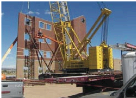
Figure 2.2-2: Prefabricated roof truss installation (Mortenson Construction, 2011)
