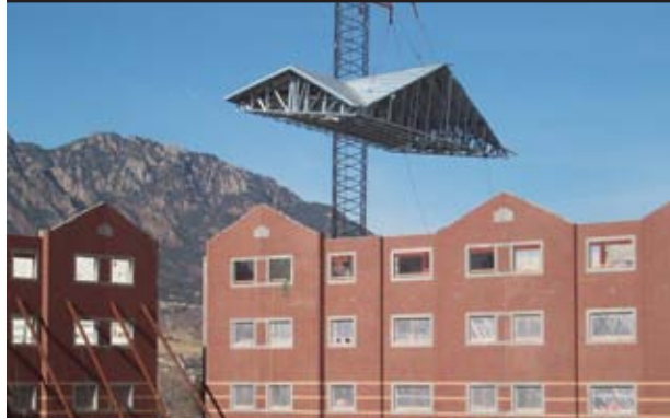
Figure 2.2-3: Precast load bearing wall panels (Mortenson Construction, 2011)
