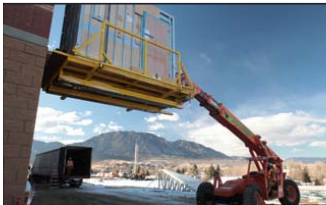
Figure 2.2-5: Pod installation (Mortenson Construction, 2011)
