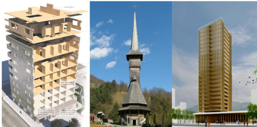
**Figure 3.1: Nine-storey Graphite Apartment building in London, constructed out of laminated wood, church of Surdesti in Maramures, Romania, 72m high known to be one of the tallest structures made out of wood, conceptual design of a 20-storey skyscraper wooden building by Michael Green.**
