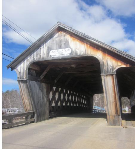
**Figure 4.4: A Town lattice truss bridge spanning over the Squam River and built in 1990 by Milton Graton and Sons.**
