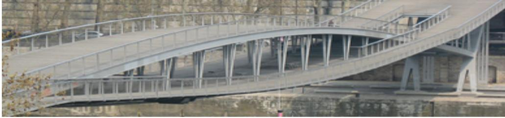
**Figure 3.21: Pedestrian bridge, Simone de Beauvoir, in Paris constructed using steel sections.**
