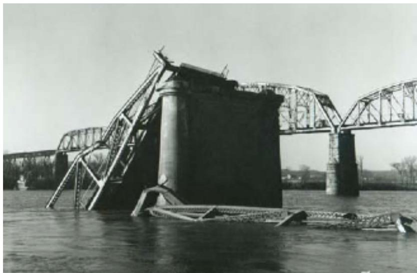
**Figure 3.22: Silver Bridge collapse in 1967 due to failure of connecting elements by corrosion killing 46 people (Zoli and Steinhouse, 2007).**
