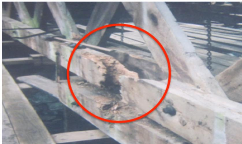
Figure 3.5: Material degradation of bottom chord of wooden truss due to biological attack that resulted in the structural failure of the truss element.
