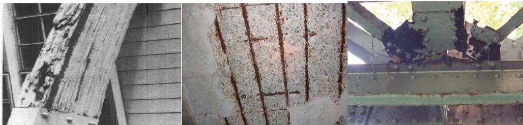
**Figure 1.1: Effect of deterioration mechanisms on the three structural materials wood, reinforced concrete, and steel.**
