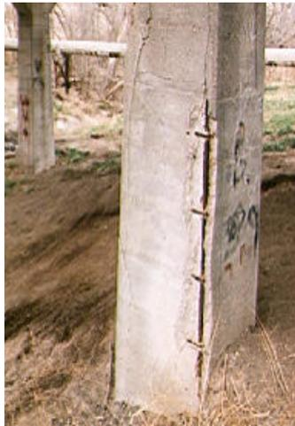
**Figure 3.17: Deterioration of a concrete pier due to corrosion of steel reinforcement.**
