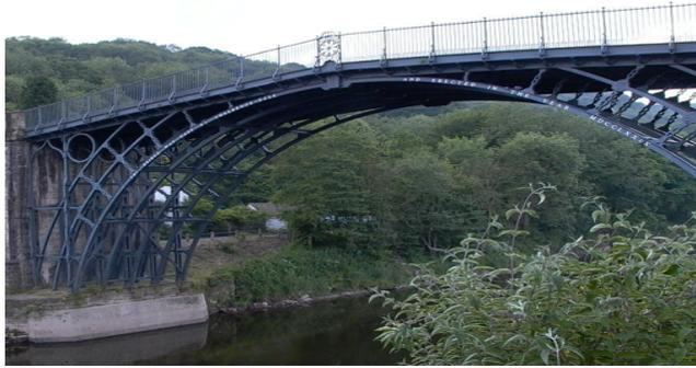
**Figure 3.20: Iron Bridge built in 1779, was the first bridge in the world constructed fully out of cast iron.**
