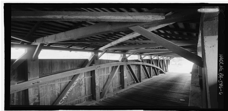
**Figure 4.3: Interior view of the Pine Grove Bridge illustrating the structural system of the Burr arch truss (Lowe, 2002a)**
