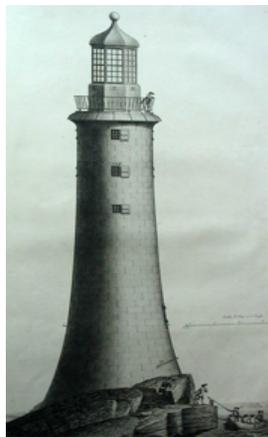
**Figure 3.11: Eddystone Lighthouse rebuilt in 1756 by John Smeaton, being the first to experiment the properties of hydraulic mortar (Mindess et al., 2002).**
