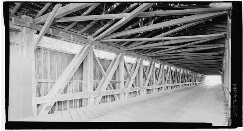
**Figure 4.6: Eldean Bridge in Troy, Ohio, illustrating the configuration of a Long truss (Lowe, 2002b)**
