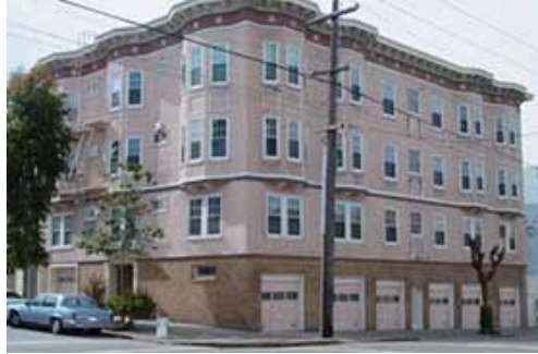
Figure 3.1.1. Multi-Family Wood-Frame Residence, San Francisco. Image courtesy of ABAG.ca.gov
