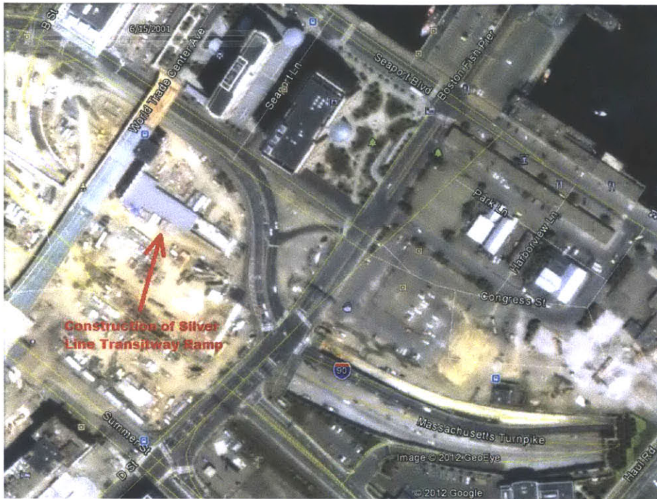
Figure 7-2: Silver Line Transitway Ramp Construction 76
