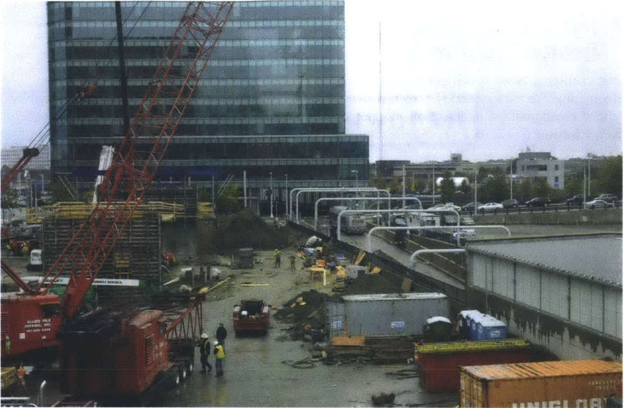
Figure 7-1: Construction of Waterside Place Development. Photo Taken on 10/10/2012
