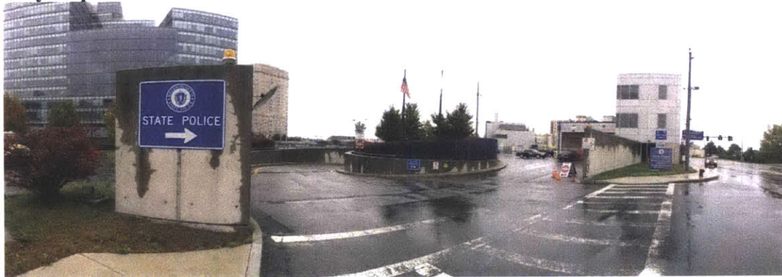
Photo 6-9: Ramp connection to Haul Road
