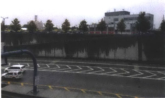
Photo 6-7: Ramp viewed from Silver Line Way stop
