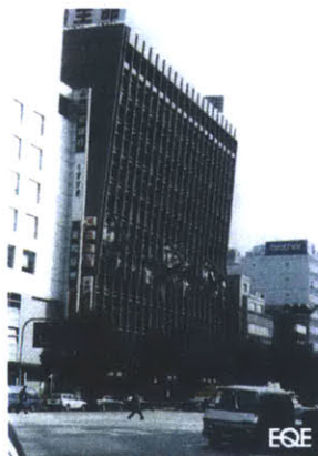
Figure 1-12: Damaged exterior columns, Kobe 1995
