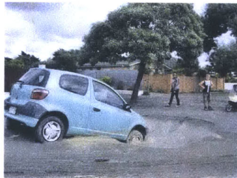
Figure 1-9: Soil liquefaction, Christchurch 2011
