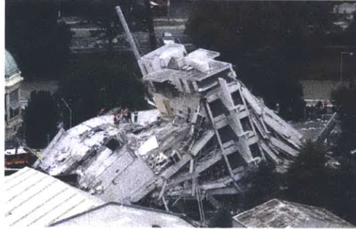
Figure 1-7: Collapsed Building, Christchurch 2011
