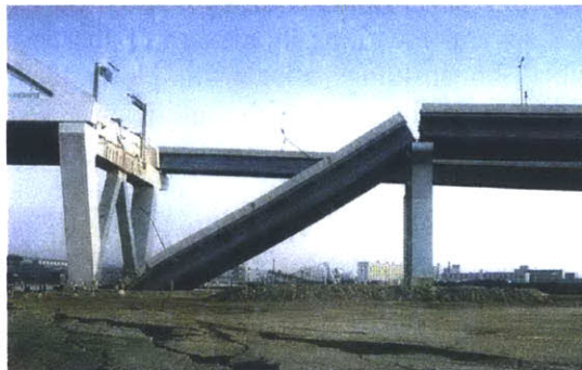
Figure 1-11: Collapsed bridge deck, Kobe 1995
