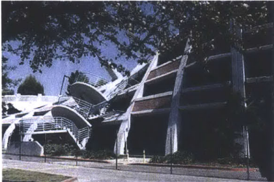
Figure 1-4: Building collapsed after the Northridge earthquake
