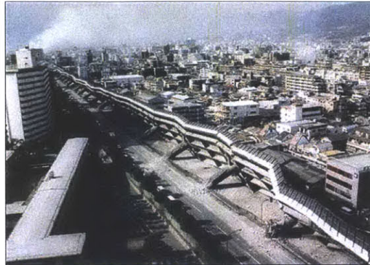
Figure 1-10: Collapsed aerial highway, Kobe 1995
