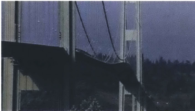
Figure 1.1 – Tacoma Narrows Bridge: excessive deformation and subsequent collapse due to resonance
