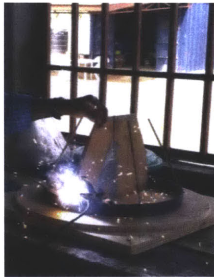
Figure 31: Welding steel rod to the base ring
