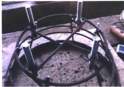
Figure 34: Metal cage, with threaded rods
