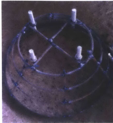
Figure 35: Finished metal cage
