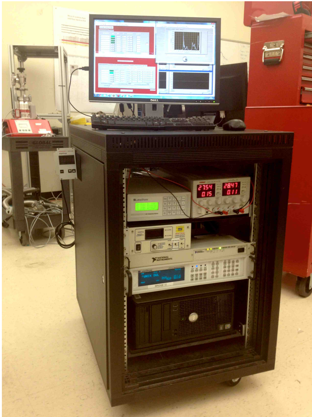
Figure 4-38: A wheeled miniature server rack houses the GSE, providing a portable control and readout platform for the instrument. The current laboratory configuration is shown, from bottom moving upward: the control computer with data acquisition and synthesis card; resistive thermometer readout; LHe level gauge; diode thermometer readout; 28 V dual power; monitor with various running GUIs.
