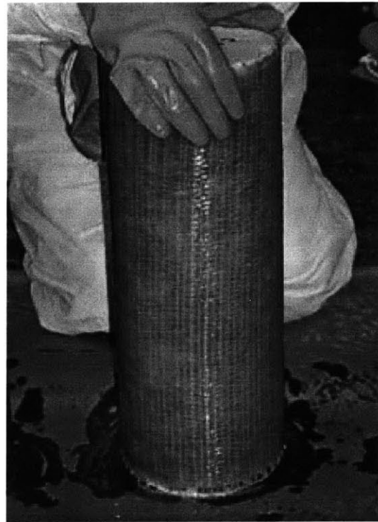
Figure 4.10 Squeezing entrapped air and ensuring a smooth finishing
