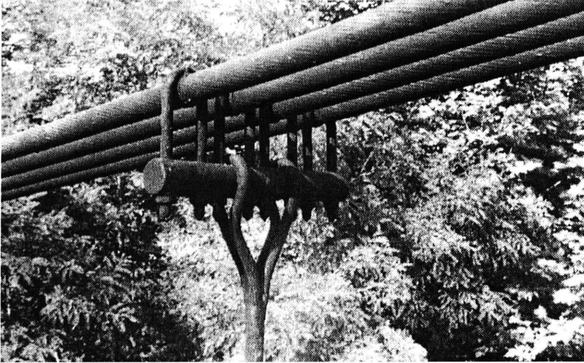
Fig. 8 Flat rectangular disposition of cables
