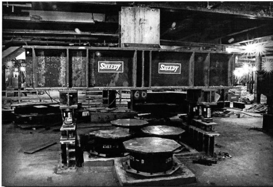
Figure 30 – Installation by Sheedy Drayage, San Francisco City Hall, CA.
