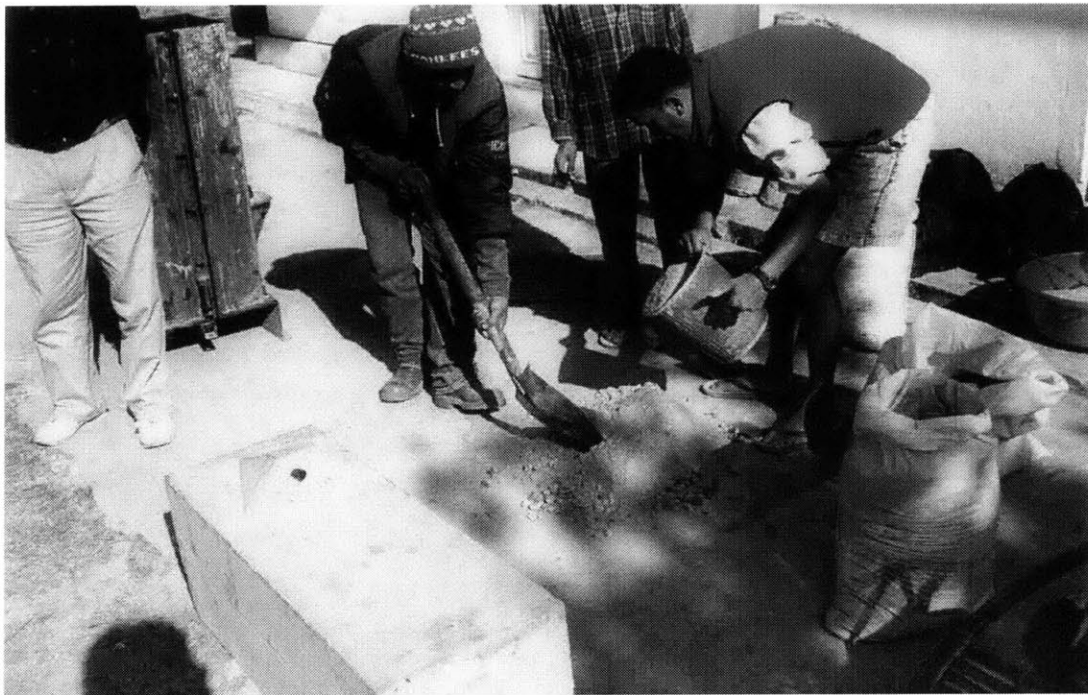
Figure 12: Concrete Mixing I
