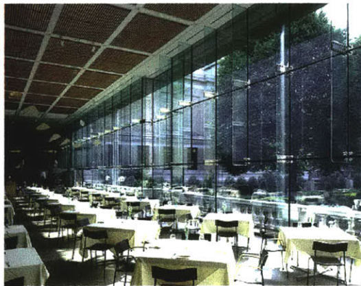
Figure 18 - Glass Fins, Museum of Fine Arts, Boston, Massachusetts (W&W Glass Systems, Inc., 2000)
