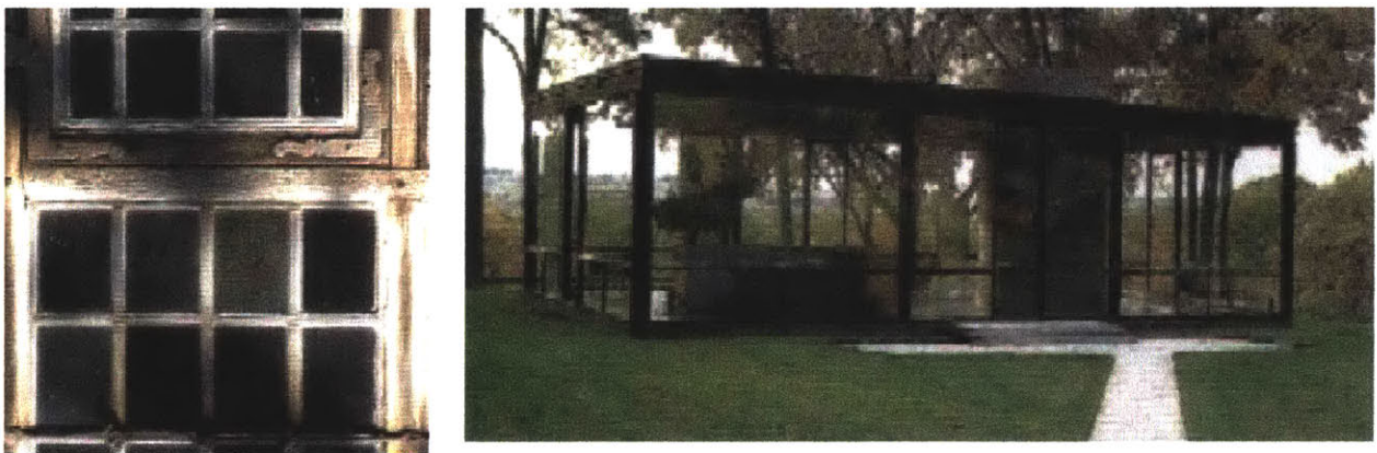
Figure 2 - Improvement in Size and Transparency from 17th Century to Modern Glass (Schittich, 1999)
