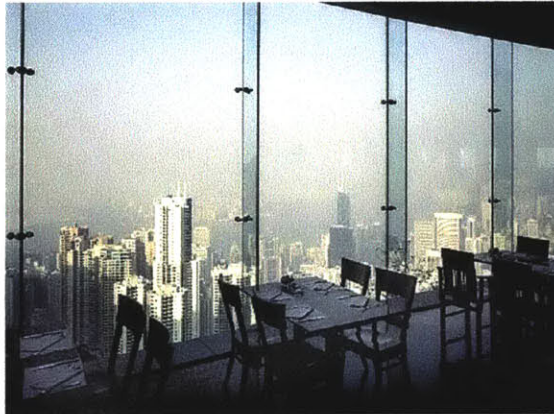
Figure 17 - Glass Fins, Park View Restaurant, Hong Kong (W&W Glass Systems, Inc., 2000)
