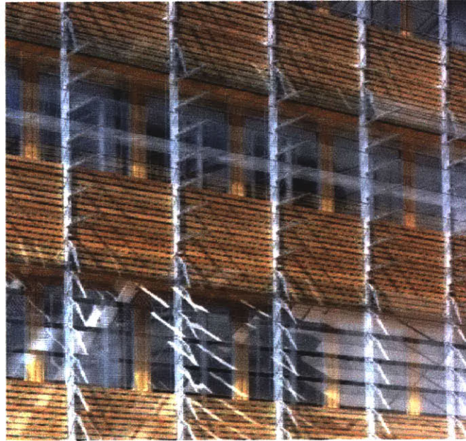
Figure 5 - Dynamic Glass Façade (Schittich, 1999)
