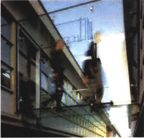
Figure 3 - Structural Glass Pedestrian Walkway (Schittich, 1999)
