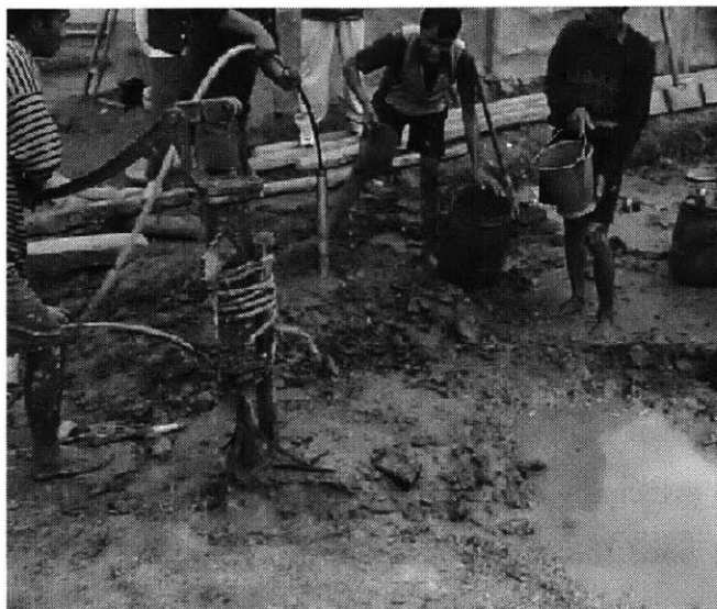
Figure 5-1. Construction of a Tubewell
