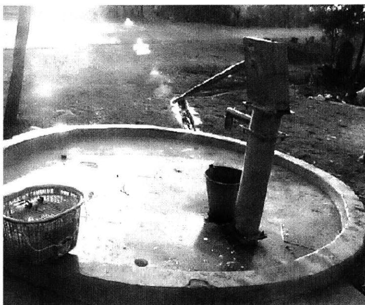
Figure 2-5. A Lift Tubewell
