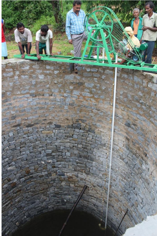
Figure 4.33. Lowering the pipes and rope into the well.
