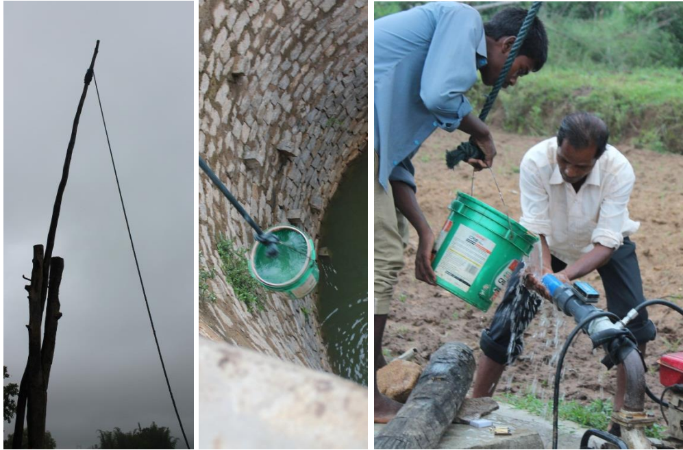
Figure 2.16. Retrieving water from the well using a counterweighted lever and priming the pump by hand.
