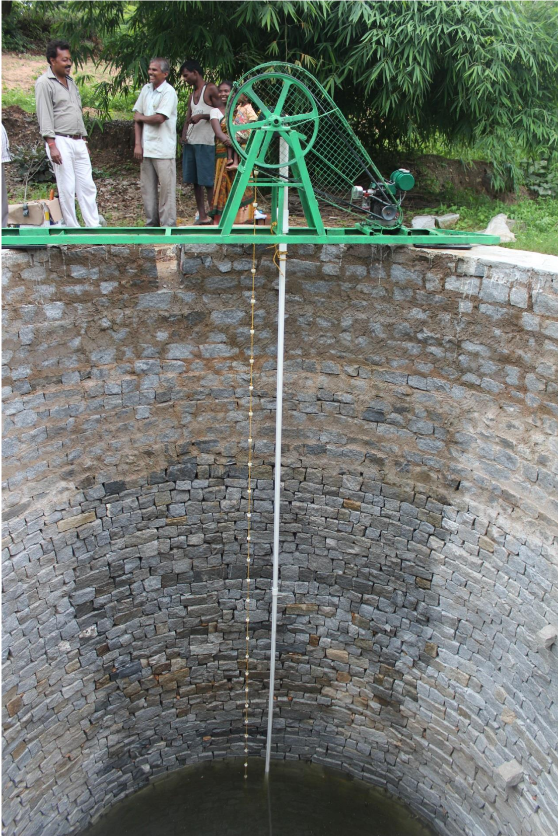
Figure 4.35. The complete installation of the rope pump on the well in Ruitola.
