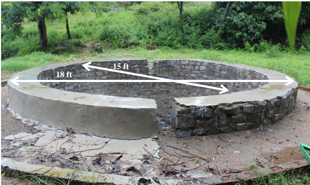
Figure 4.30. Well in Ruitola village used for the rope pump trial.
