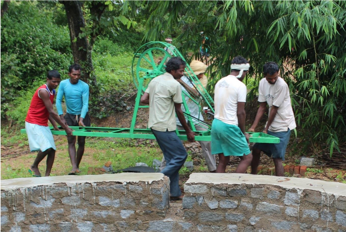
Figure 4.31. Carrying the pump to the well.
