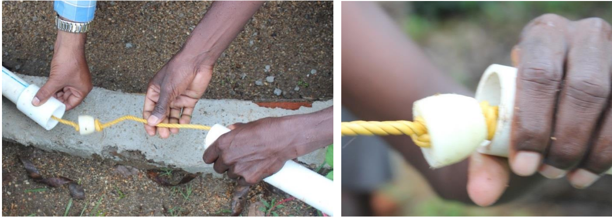
Figure 4.32. Inserting the piston into a pipe, narrower side inwards.
