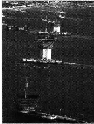
Fig.13: All piers in their final position (source: www.gefyra.gr )
