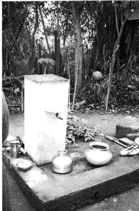
Figure 11: Arsenic-Biosand filter in the backyard of a house in Sarawal
