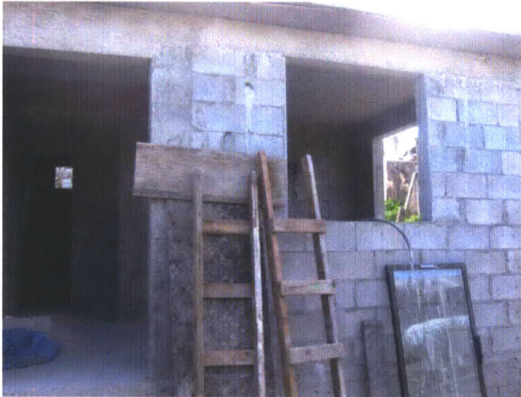
Figure 3.13 Construction progress, exterior
