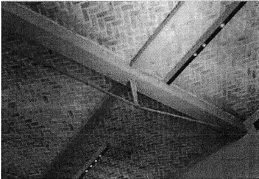
Figure 4.9 Tile domes with iron beams and ties
