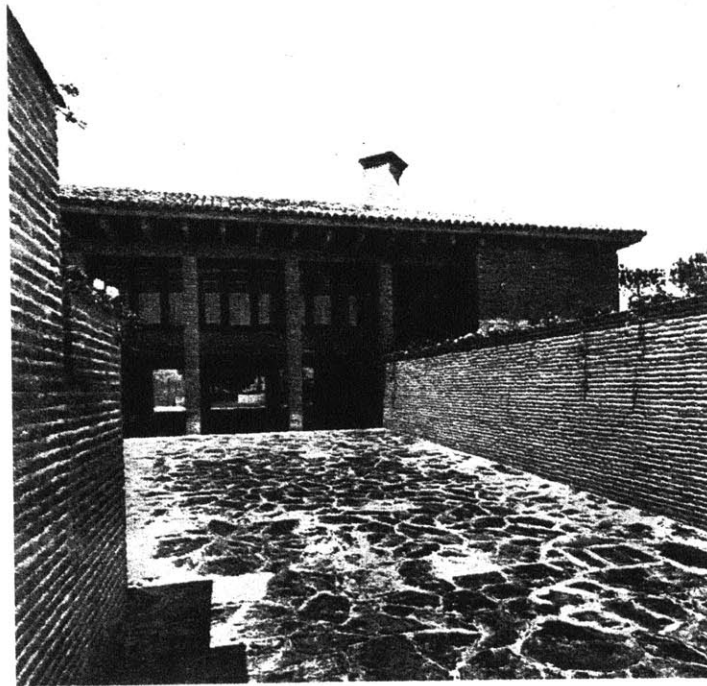
Fig. 29 House Gómez-Acebo partial view of south façade
