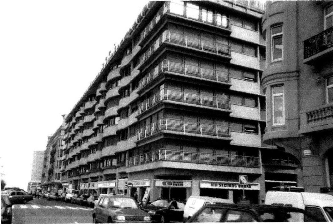
Fig. 41 Urumea Housing, exterior view
