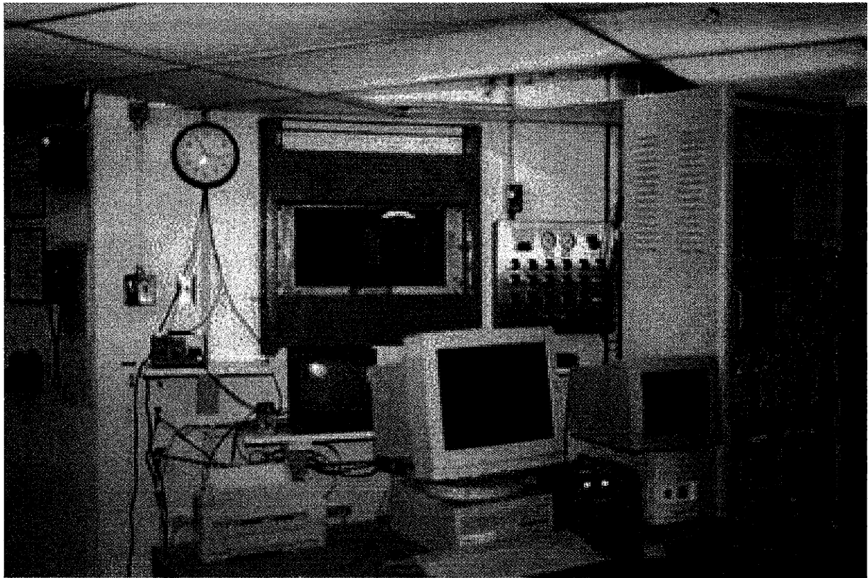
Figure 4.5: Medical area outside the MITR-II M67 medical therapy room. The therapy room can be seen through the window in the center of the picture. The shutter controls are located on the panel immediately to the right of the window. Photo Courtesy of http://web.mit.edu/nrl/www/
