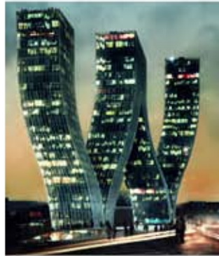
Fig. 37 BIG Walter Towers [Unbuilt] - Prague, Czech Republic
