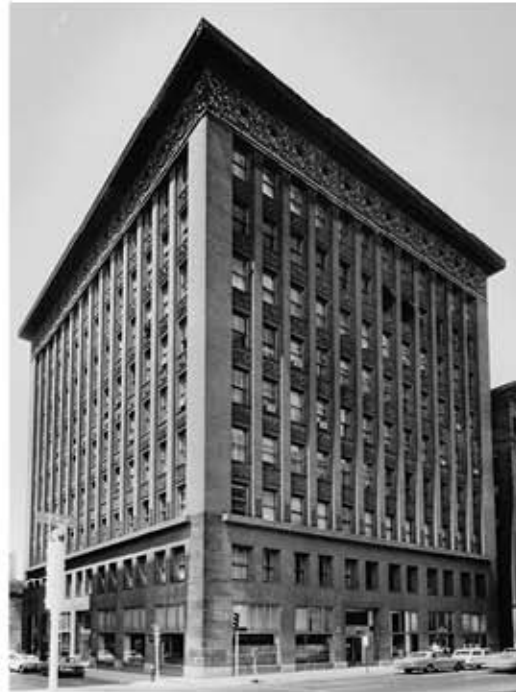
Fig. 4 Wainwright Building, (1891), St. Louis by Adler & Sullivan
