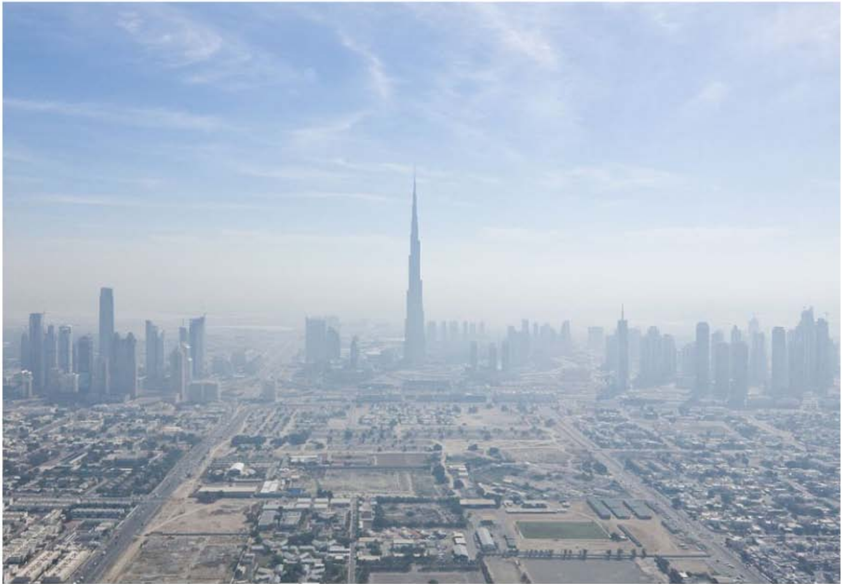
Fig. 28 View of Burj Khalifa in Dubai, United Arab Emirates.
