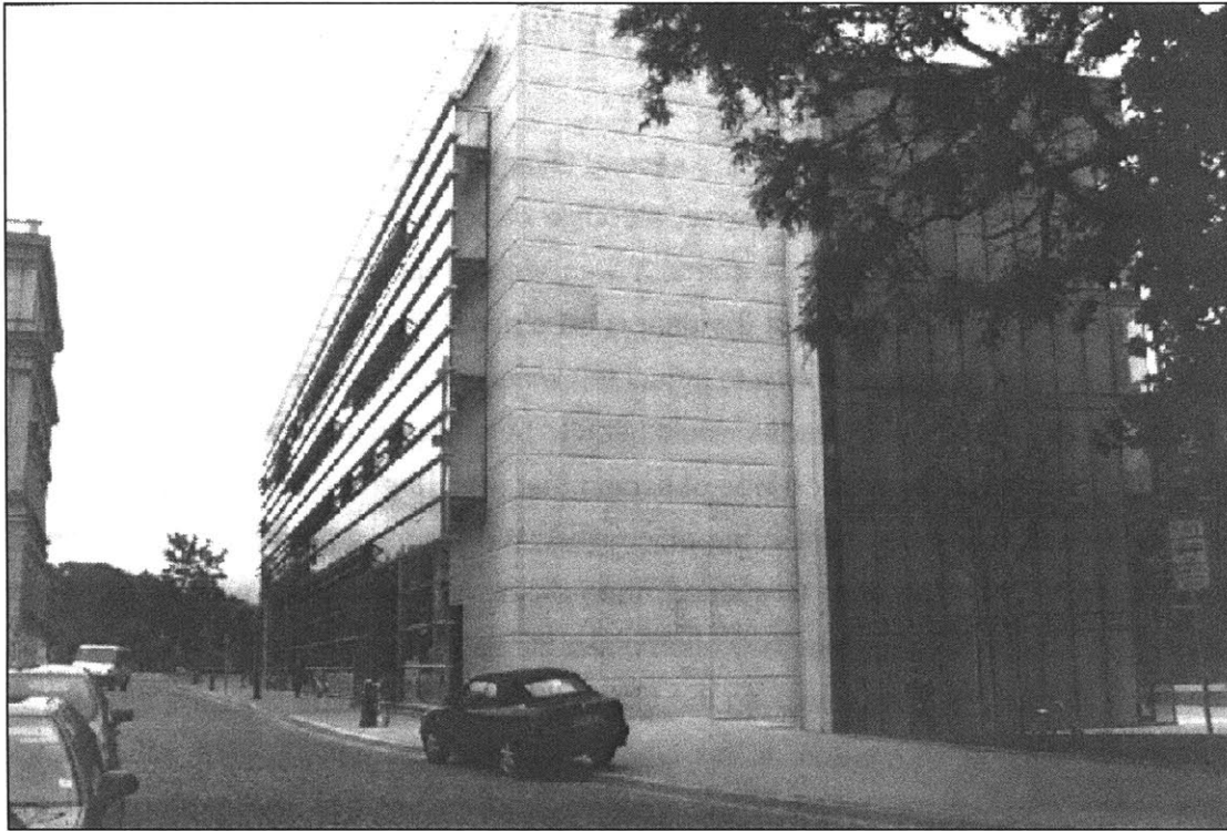
Figure 22 View of Max Planck Gesselschaft: double-skin facade protrudes from building mass. Flap windows in open position are visible.
